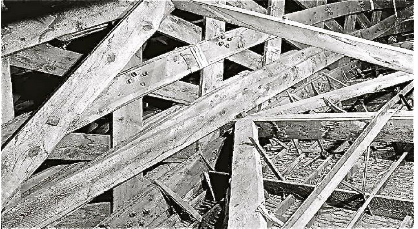
Timbers supporting Tabernacle Ceiling
